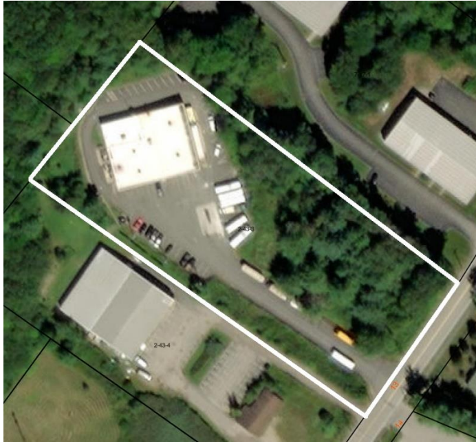
Figure 6 Aerial View Showing 13 Pomerleau St. Property Lines (Source: BiddGIS)
